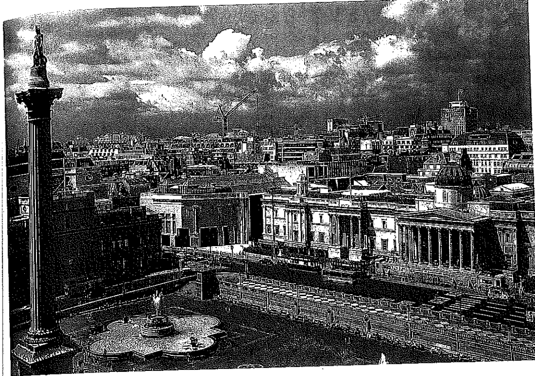
25.5 Robert Venturi and Denise Scott Brown, National Gallery, London, with Sainsbury Wing visible left of the main gallery across Trafalgar Square. 1987–91.
