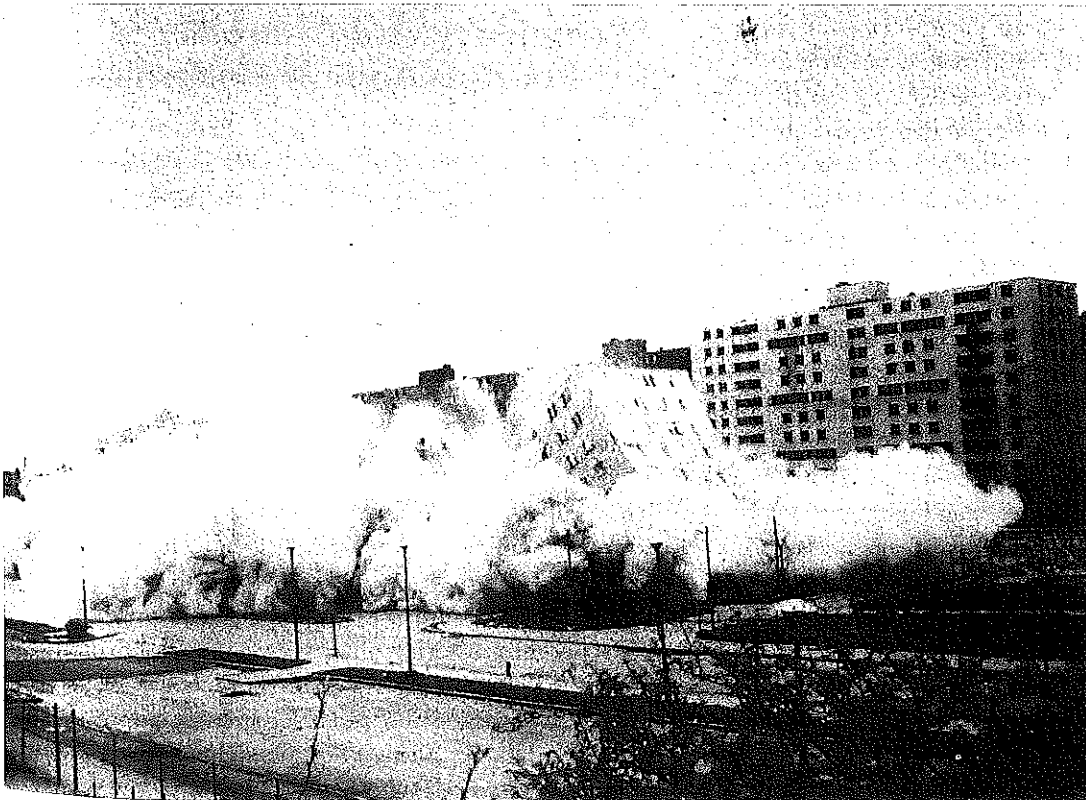
25.1 Minoru Yamasaki, Pruitt-Igoe public-housing project, St. Louis, at the moment of its demolition on July 15, 1972. Built 1952–53.
