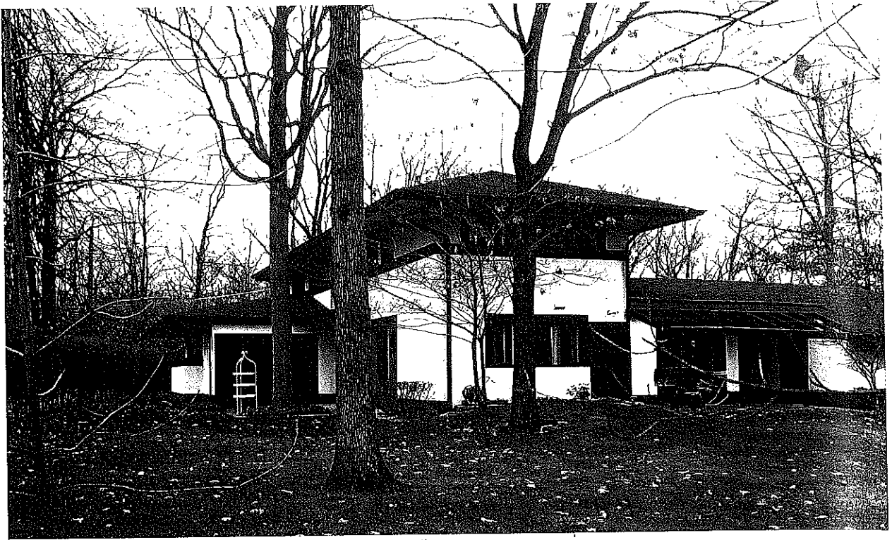
12.1 Frank Lloyd Wright, Ward Willits House, Highland Park, Illinois, 1902–3.
